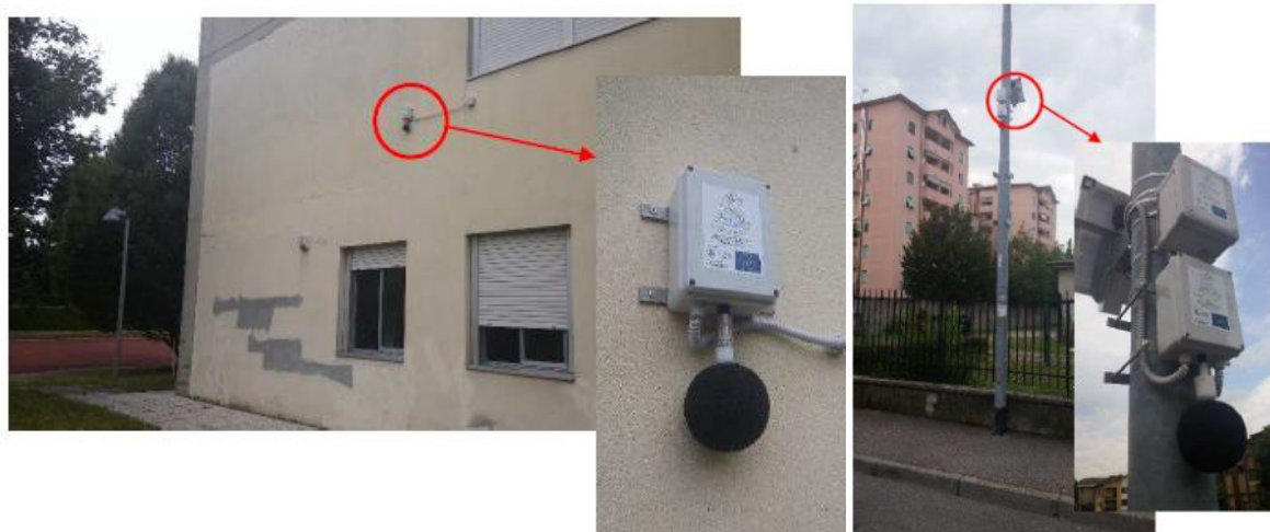
Figure 22 – The installation of the system in the public building façade (left) and light pole (right) [31].
